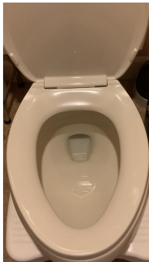
Post test— leak fixed
