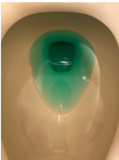
Parent's toilet — leak detected
