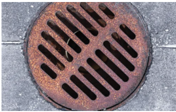
I ♥ Storm Drains
